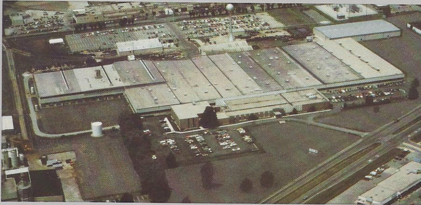
Main offices and plant, Concord Road
