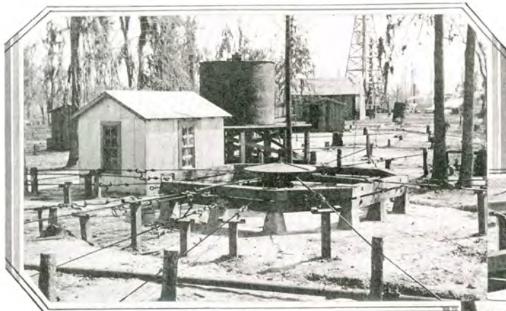
SUN COMPANY INSTALLATION LIBERTY, TEXAS
