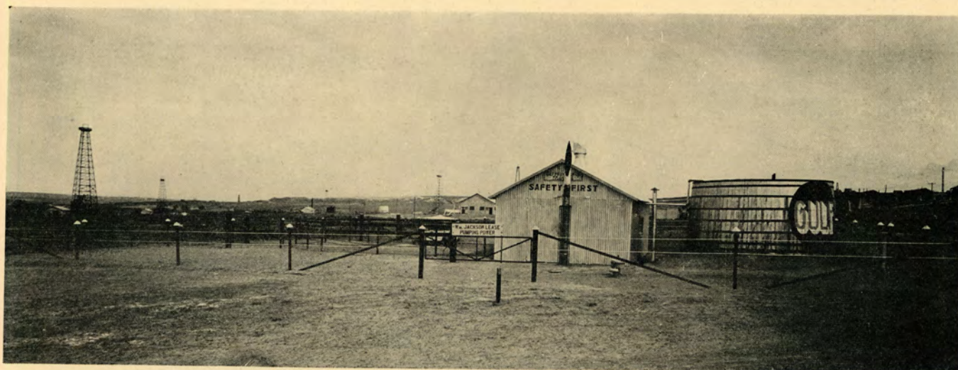
The First Central Power Installed in Grey County, Texas
