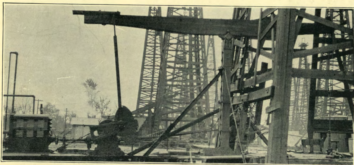
Vacuum Lease, Liberty, 3500 feet—One of our original units installed with beam balance making 28 strokes, as fast as rig could go, without "whipping" balance weights. Later, when rig was equipped with Trout counter-balanced crank, strokes were increased to 36 in out hole.
