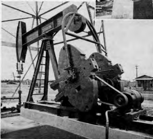
Figure 13 HUMBLE OIL & REFINING CO. Lufkin Double Reduction Twin Crank Unit driven by electric motor.
