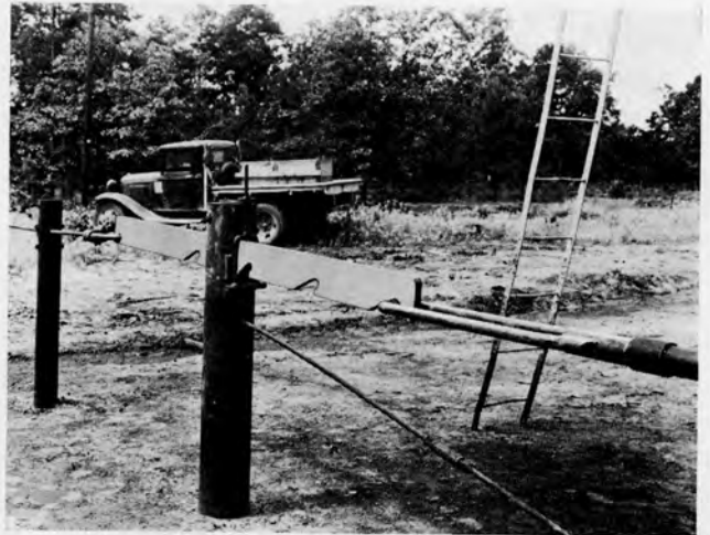
Figure 54 Lufkin "slide bar" type knockout renewable oak filler block with positive "hook-off" arrangement.
