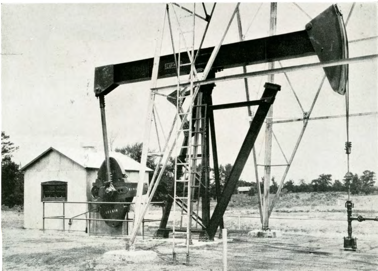
FIGURE 41—Typical Lufkin Single Crank Unit installation
