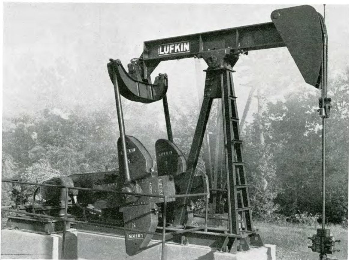
TC-55-7A with Trout simplified cranks. 42" stroke.
