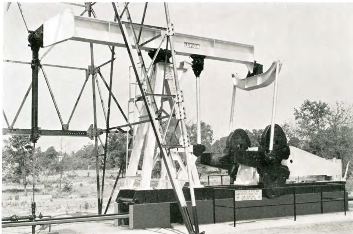
Above: All Lufkin Units (Except 66-5 and 77-3) are arranged to apply Bell Crank for pumping extra wells.
