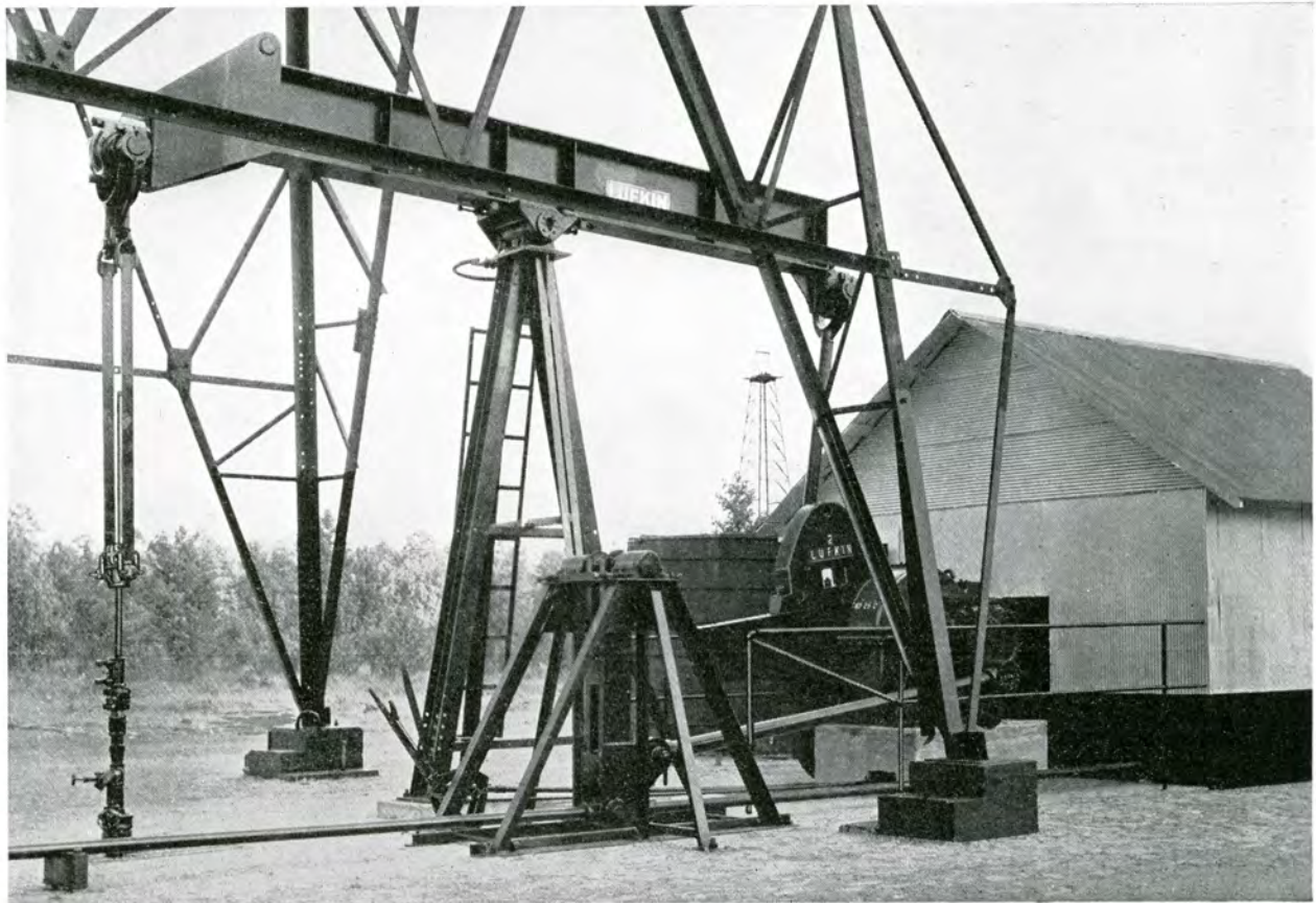
Bottom: Similar installation of heavier type with Universal Hanger and double channel single arm take-off pumping two additional wells.
