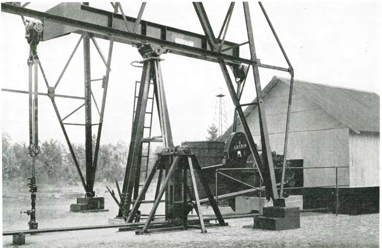
Bottom: Similar installation of heavier type with Universal Hanger and double channel single arm take-off pumping two additional wells.
