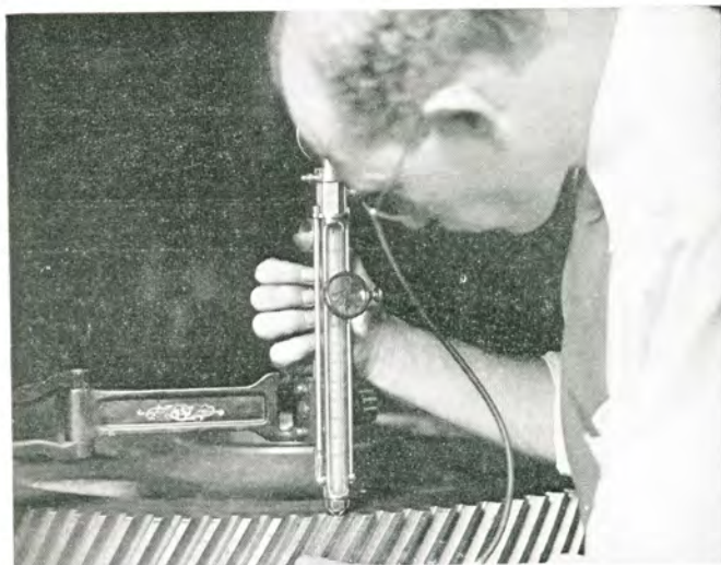
Testing Gear Teeth for Hardness.
