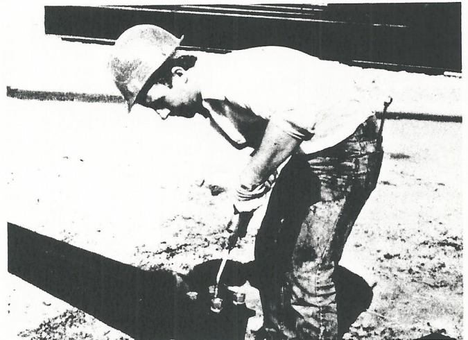
Figure 12 — Lubricating upper pitman box.
