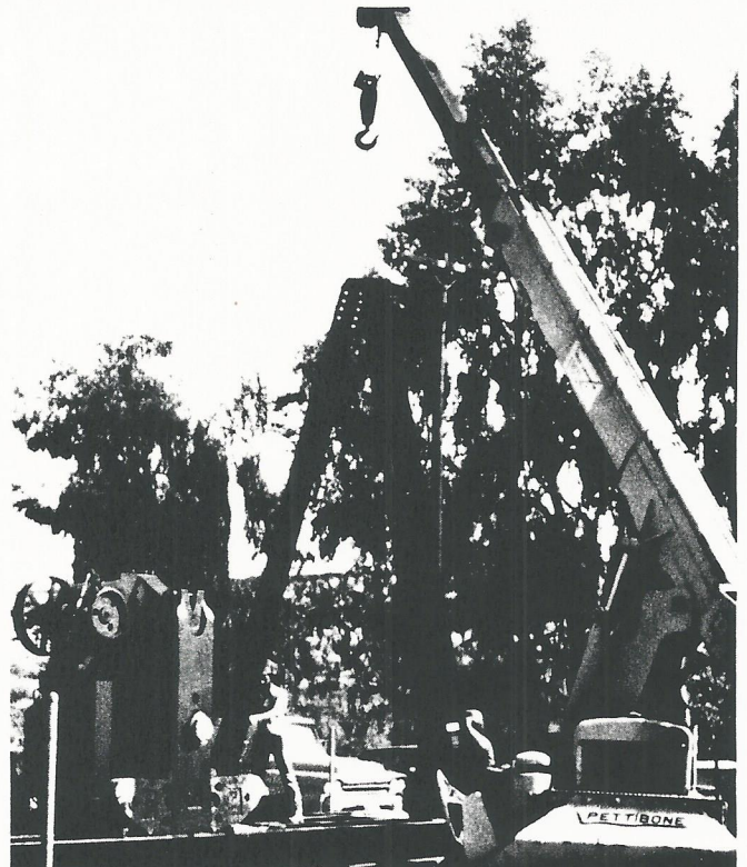
Figure 9 — Installing samson post.
