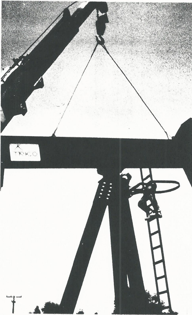
Figure 14 — Securing center bearing to samson post.
